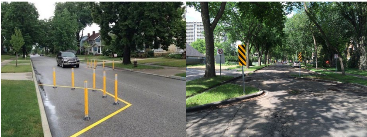
Figure 4: Chicane Treatments (Left – Low Cost Quick Build Option; Right – Permanent Feature with adjusted Curb Line) (Source: City of Edmonton - Community Traffic Management)
