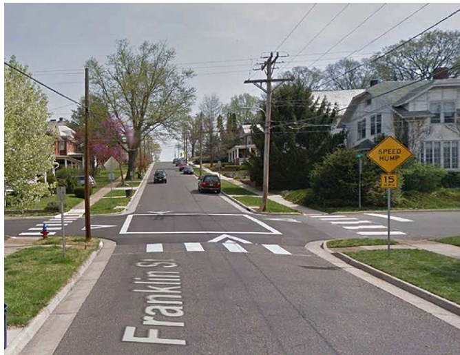
Figure 10: Raised Intersection (Source: FHWA Traffic Calming ePrimer)
