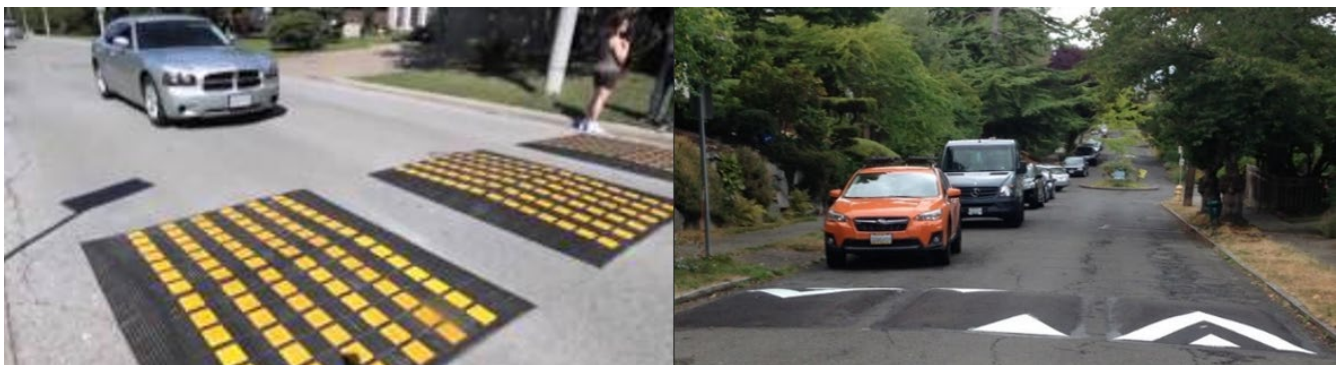
Figure 5: Speed Cushion (Left – Temporary Speed Cushion Mats; Right – Asphalt Speed Cushions) (Source: Google)
