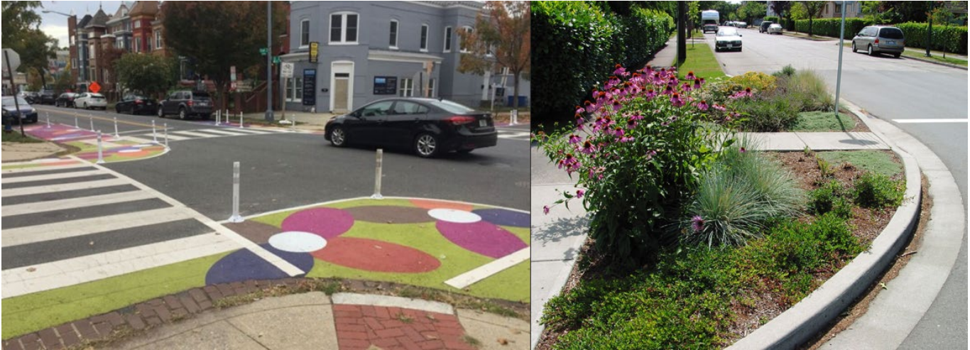
Figure 8: Curb Extensions (Left – Painted Blub-outs; Right – Permanent Landscaped Curb Extension) (Source: Google)
